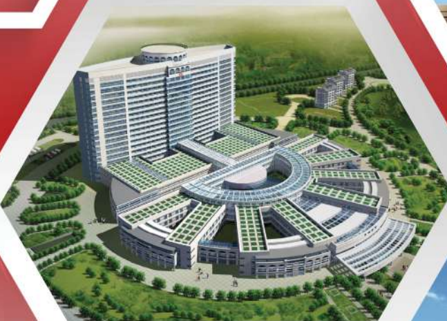
Fujian Shishi People's Hospital
